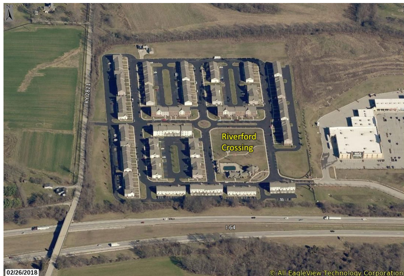
Figure 14: Riverford Crossing Apartments
